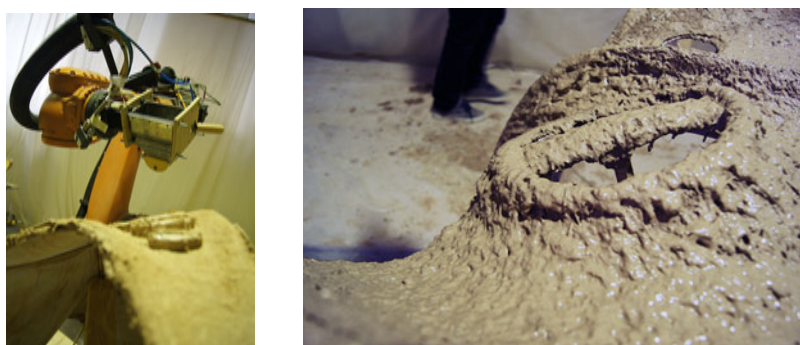
Figure 7: Concrete hand sprayer “Sablon” connected to Kuka robot with fibrous mix spraying on the earthen shell in progress. Iaac seminar May 2016. [Photos by the seminar’s participants].
